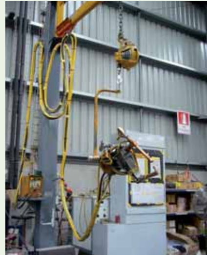
Welding equipment on counterbalances.
